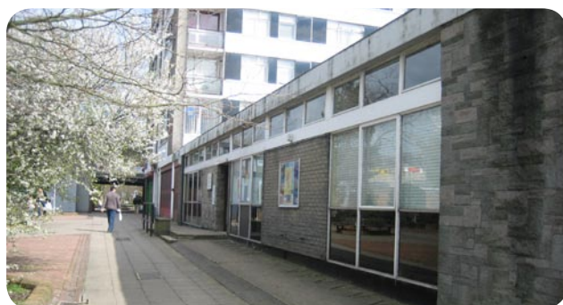
Figure 2: Hatfield Library before refurbishment Photo: Bryden Wood Associates
